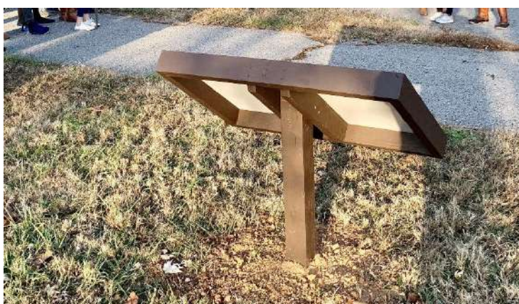
Photo 2: 2x4s run along the back of the panel frame and attach to the 4x4 post; the bottom of the frame is about 18" from the ground.
